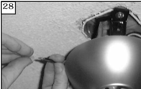
28 Make wire connections to power source using wire nuts provided. Make sure that no filaments are outside of the wirenut. After making the wire connections, the wires should be spread apart with the grounded conductor and the equipment-grounding conductor on one side of the outlet box and ungrounded conductor on the other side of the outlet box.
